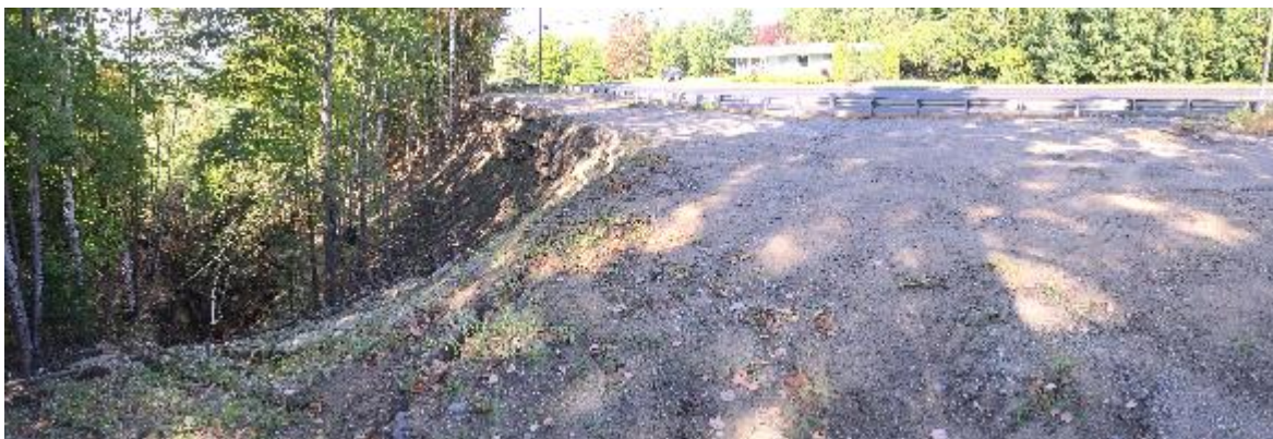
Figure 18: Photo of the head of the gully (filled in and curbed).
